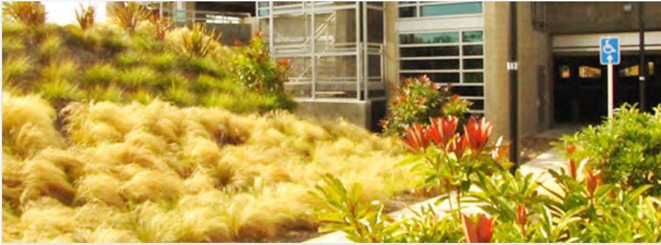
The four-level Parking Structure and Police Substation provides parking for 1,200 cars.
